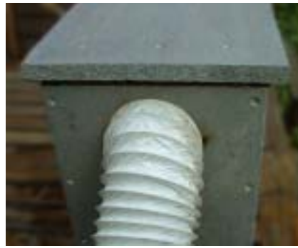
The outlet end of the box showing the plastic flexible ventilation pipe.
